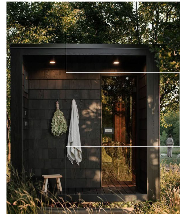
3.A discreet private entrance sets the stage, offering a glimpse of the experience awaiting inside. Strategic lighting guides guests, complementing the dark timber-clad frontage.
